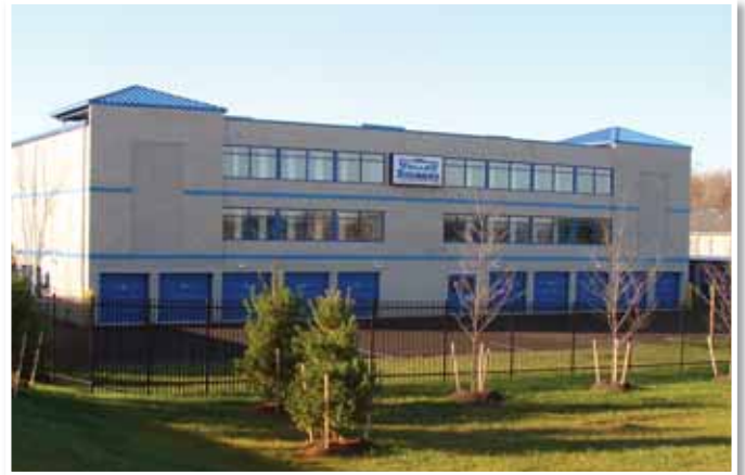
To maximize his site, this owner has one large three-story building and two single-story buildings with no interior hallway.
